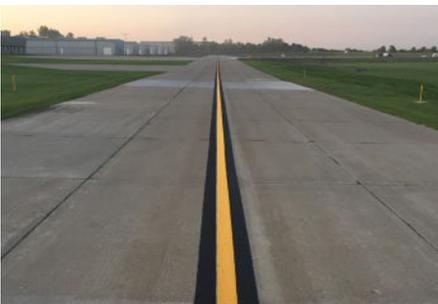
The scope of the project included removing and replacing the existing concrete pavement of Taxiway A and C North with 8 inches of PCC pavement underlain with 6 inches of aggregate base course placed on 12 inches of cement treated subgrade. Edge lights affected by new pavement construction and updates to fillet geometry were salvaged and re-installed on new bases. Taxiways B, C, & T-Hangar Taxilanes were rehabilitated using partial depth and full depth PCC patching and slab replacement methods.
