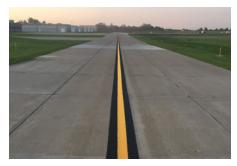
The scope of the project included removing and replacing the existing concrete pavement of Taxiway A and C North with 8 inches of PCC pavement underlain with 6 inches of aggregate base course placed on 12 inches of cement treated subgrade. Edge lights affected by new pavement construction and updates to fillet geometry were salvaged and re-installed on new bases. Taxiways B, C, & T-Hangar Taxilanes were rehabilitated using partial depth and full
